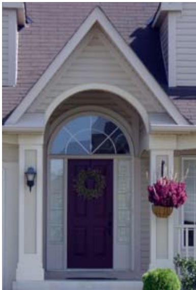
Figure 3.5a: The main entrance to the dwellings should be designed as a focal point
