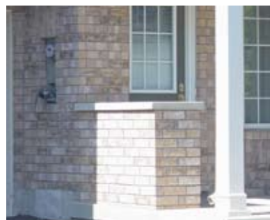
Figure 3.13c: For Townhouses, meters should be architecturally integrated or screened
