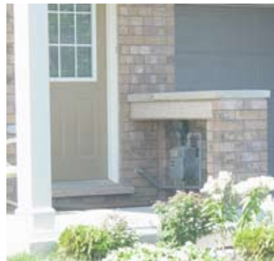
Figure 3.13a: Utility meters should be located in the interior side yard away from street view
