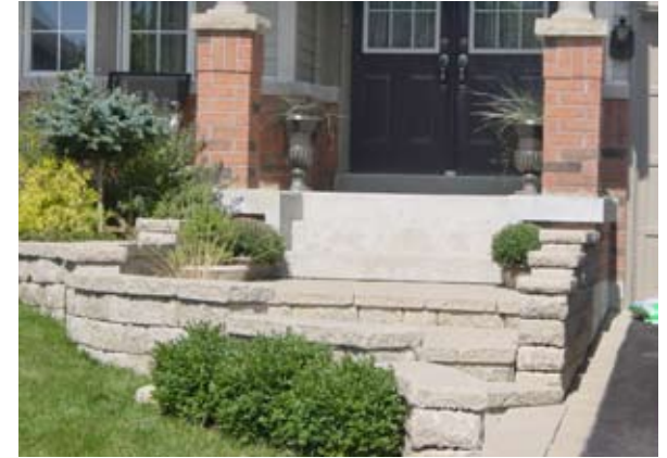
Figure 3.5b: Stairs should be designed as an integral component of the dwelling's façade
