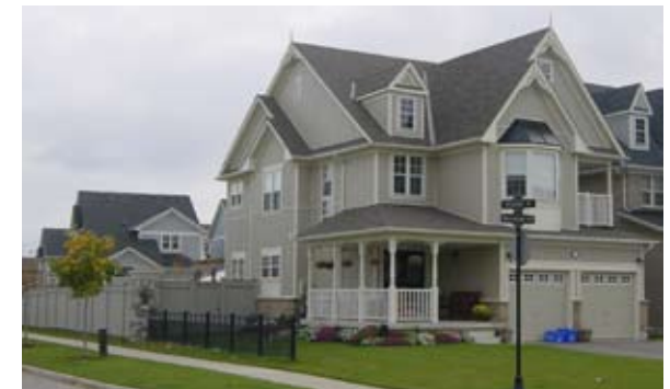
Figure 3.7.1: Image of a primarily siding-clad dwelling
